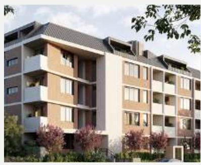
Strathfield - Pillar Projects
